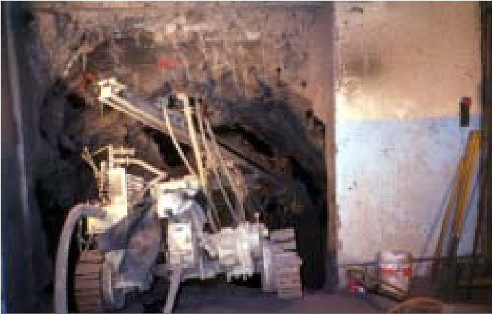
Drilling by-pass through rock
