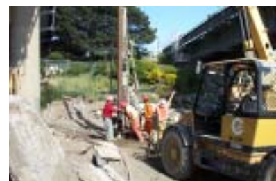
Setting 8 5/8"Ø Steel Reinforcement
