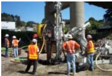
Installation of Verification Pile
